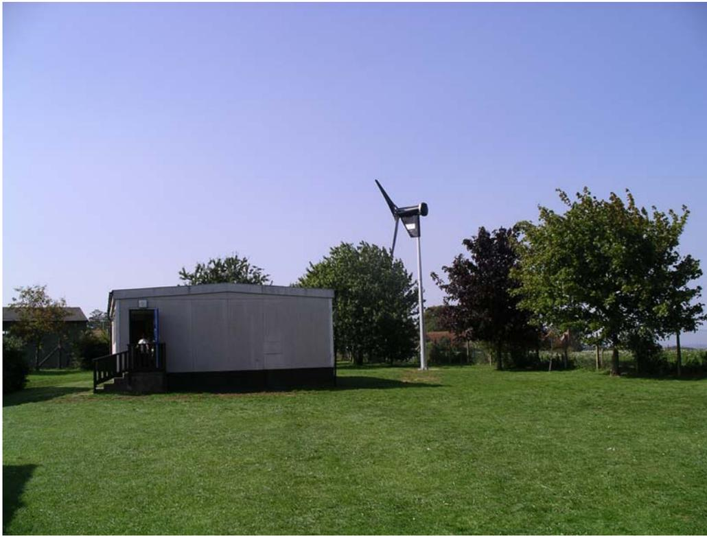
The Proven WT6000 turbine was installed 24<sup>th</sup> August 2004. The energy output recorded for two of the days since connection has been 24 and 69kWh for each day. If these figures are representative of output generally, annual generation will be between 15 and 25MWh, comparing well with the original Proven estimate of 19MWh from Proven given the average wind speed expected in the area.
