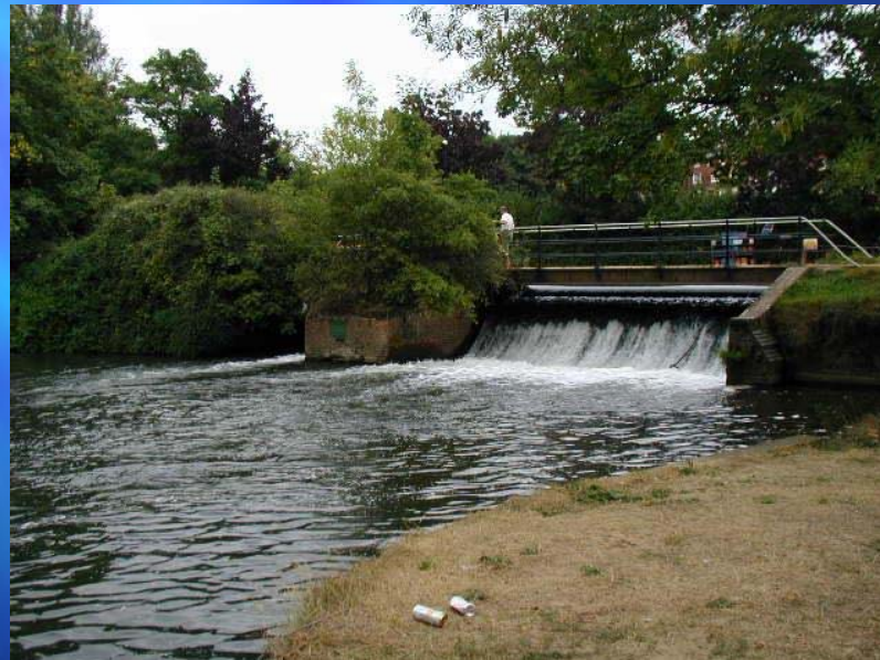
Boathouse weir and sluices - 2 & 3
