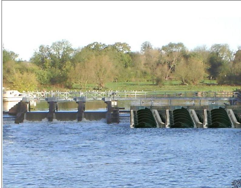
Goring and Streatley weirs next to the lock-keeper's house with photomontage of three 3.5m diameter Archimedes Screws
