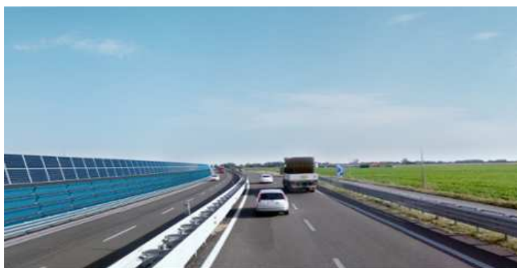
Figure 1, 1.7km PV noise barrier in Italy
