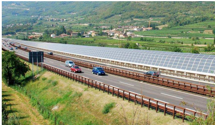
Figure 5, Italy's longest PV Noise barrier
