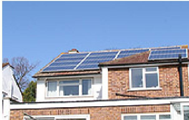
Figure 1: A domestic Solar PV system
