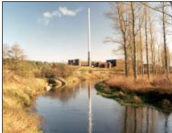
Figure 3: Thetford Power Station
