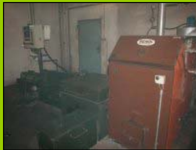
Figure 3b: 114kW Wood Chip Fired Boiler
